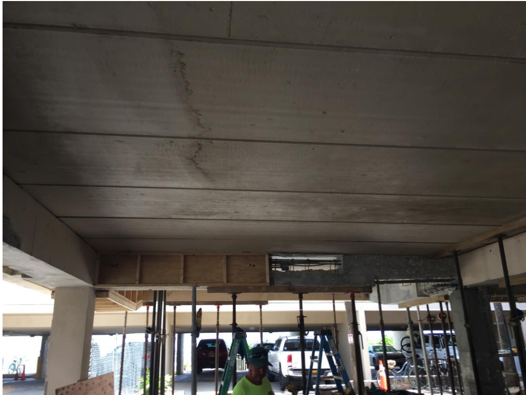
Picture 2: In-progress forming
