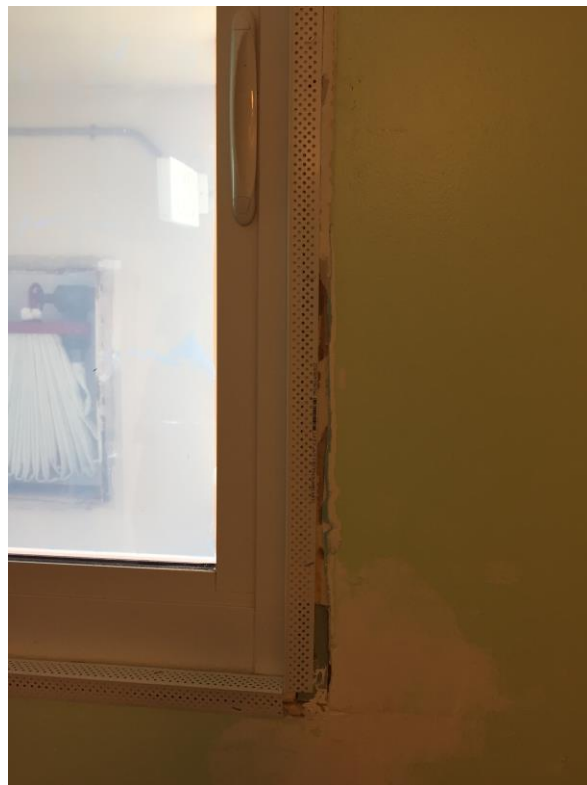
Picture 4: In-progress drywall repair
