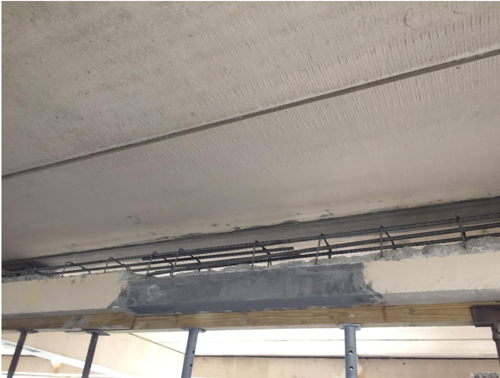
Picture 1: Approved beam excavation
