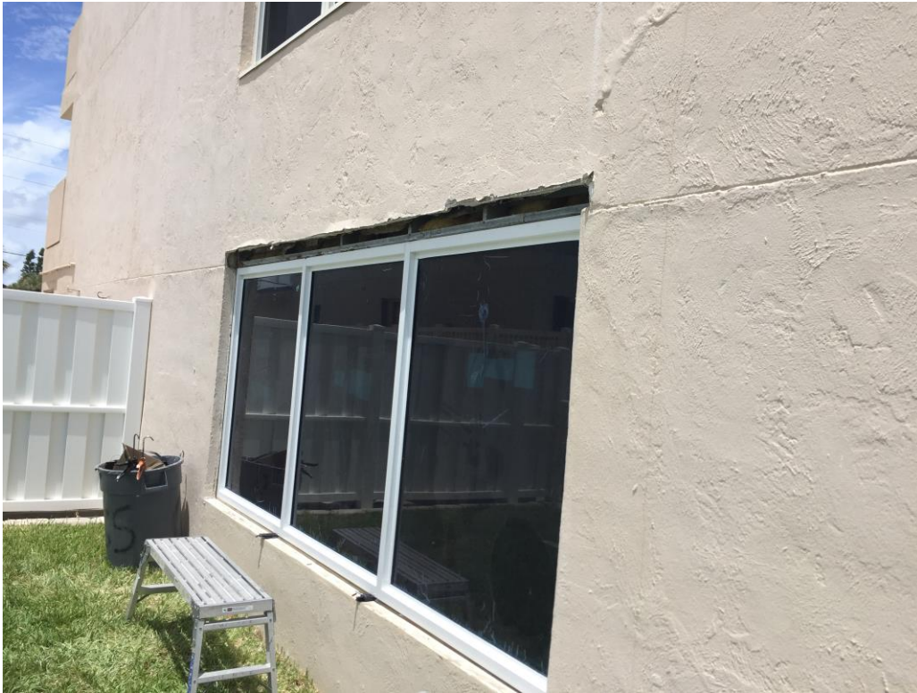
Picture 3: South elevation community room window in-progress installation
